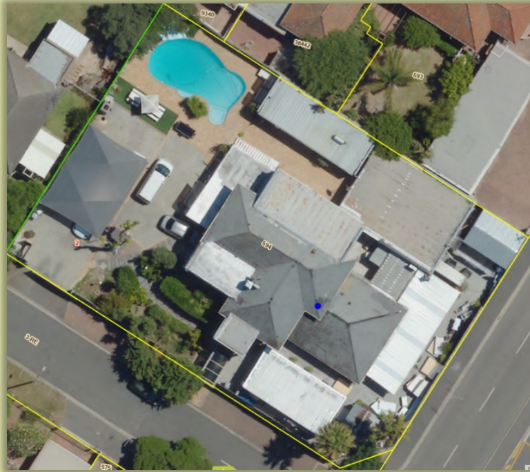
Figure 2 shows an aerial view of the subject property as it currently stands (including all the unauthorized construction). Refer to Figure 2 for clarity on the unauthorized buildings)
