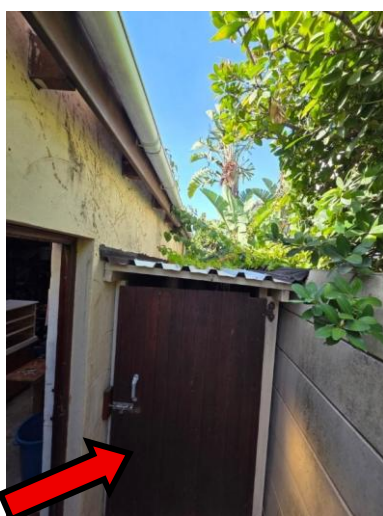
Store room on ground floor, on the eastern common boundary, behind the garage
