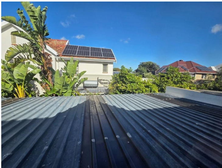
The view from the 2 nd storey games rooms window towards the east (Erf 96950)
