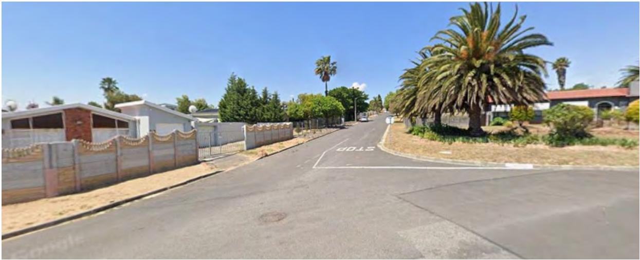
Photo 12: View looking east down Eikenhof Street
