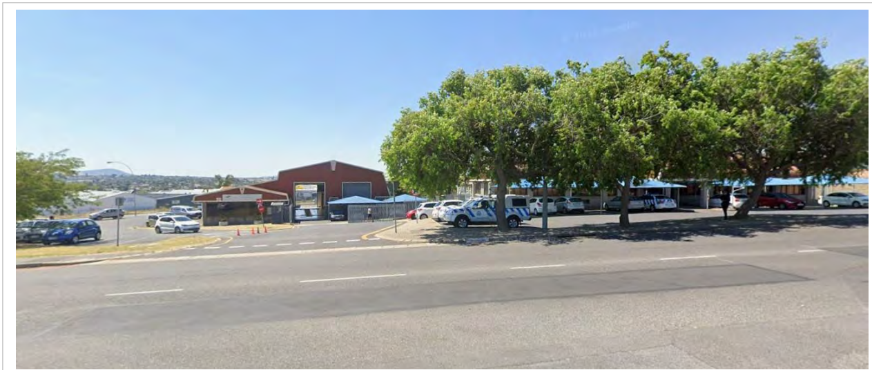
Photo 6: View looking north from Reservoir Street looking towards the Brackenfell Traffic Department.
