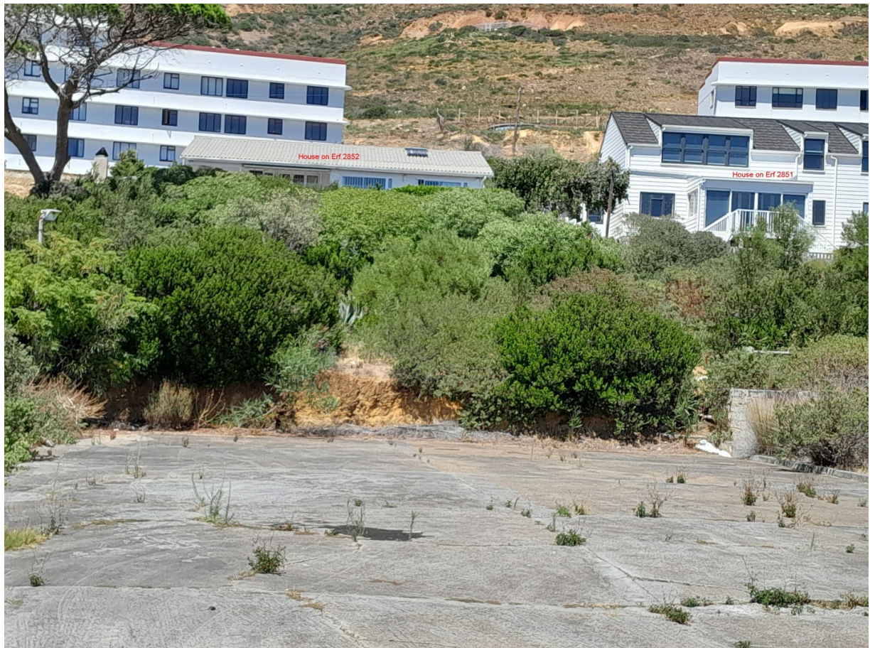
View from the Remainder towards the south showing vegetation on the vacant part of the Property.
