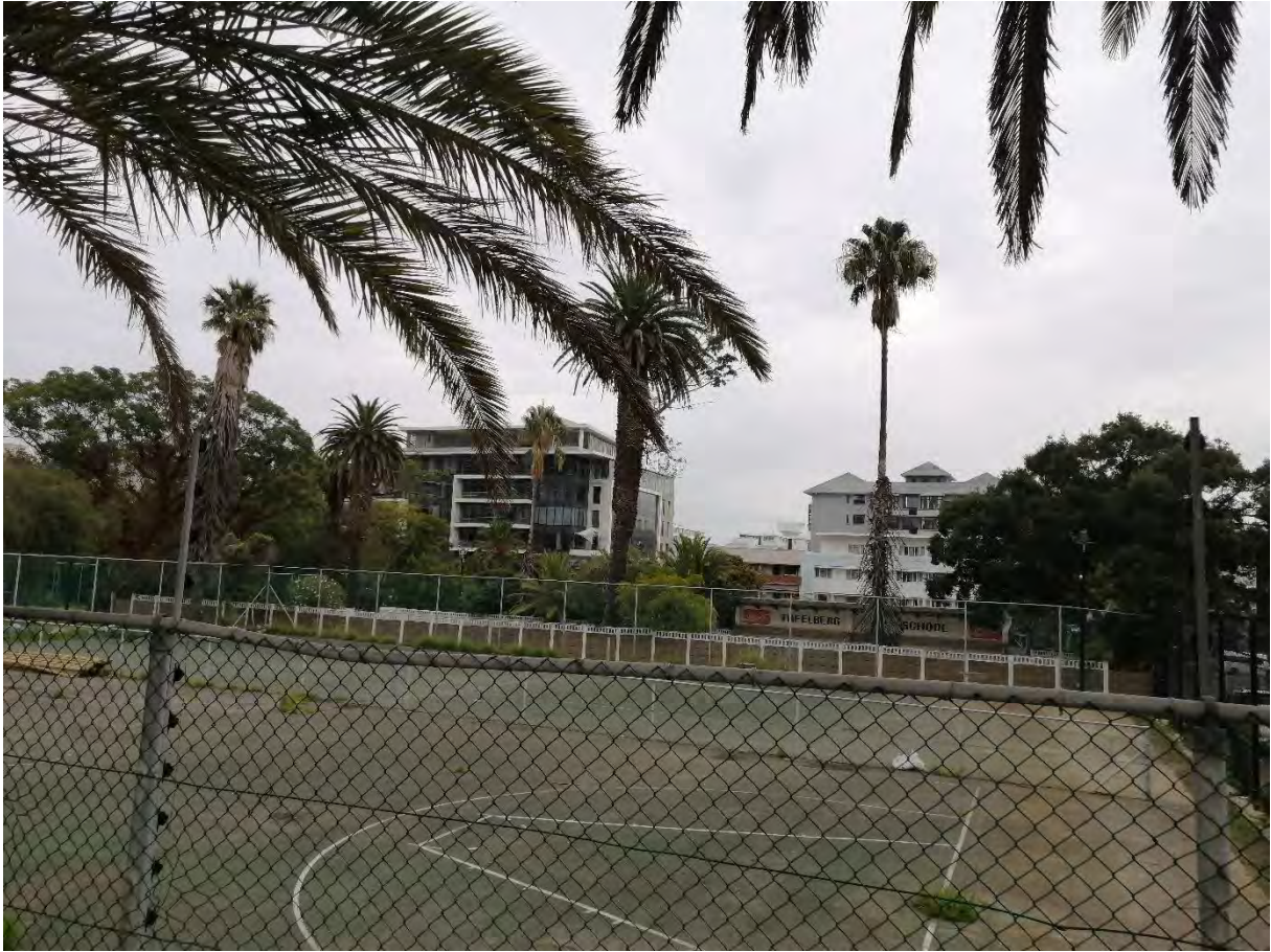
Figure 18: Abandoned Sports Facilities on the Land Portion Earmarked for Development
