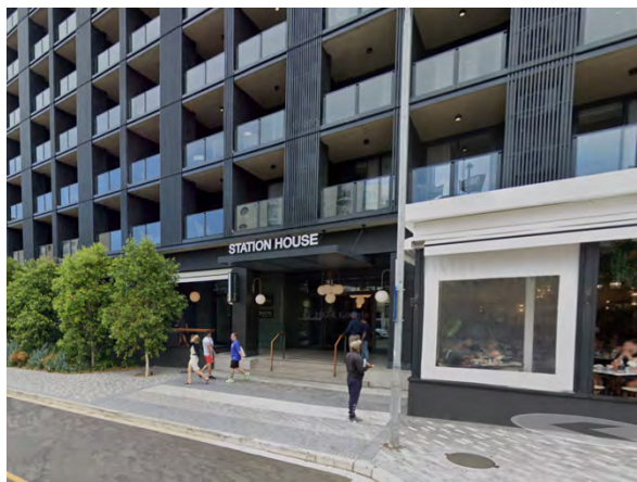
Figure 2-6 Active ground floor with residential units above. (19 Kloof Road, Sea Point).
