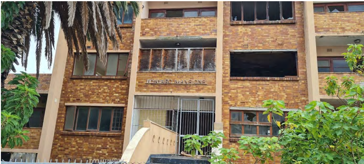
Figure 21: Abandoned Wynyard Mansions Building – Recommended for demolition – as approved by HWC
