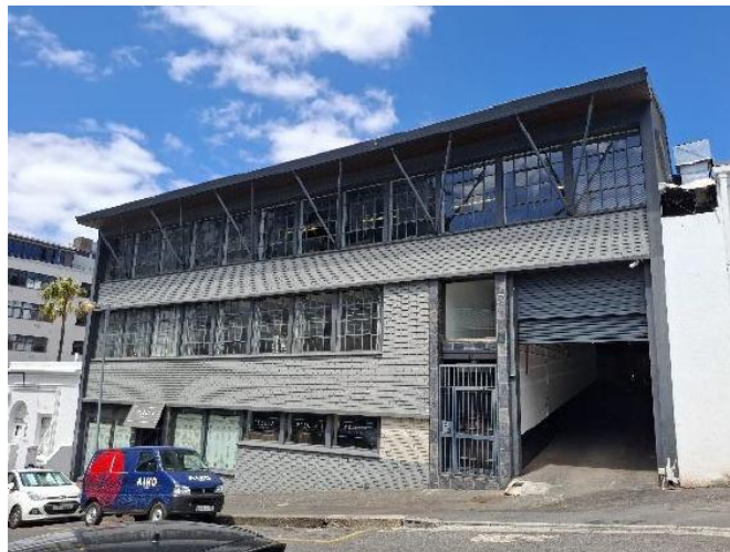
The Buiten Street façade of the property
