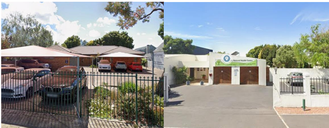
Fig. 9 & 10: Medical Offices on Erven Re548 and 459
