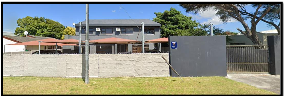
Fig. 2: Street View from Langenhoven Street
