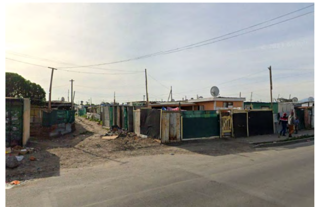
Figure 3.10: Existing informal structures – Sheffield Road / Sinqolamthi Road intersection looking east
