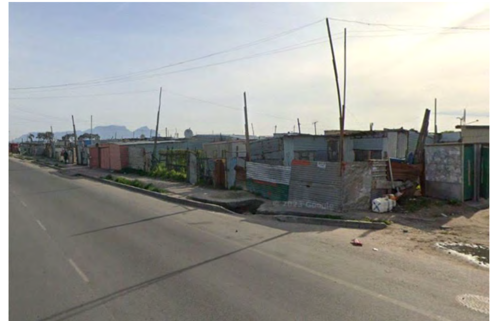
Figure 3.9: Existing informal structures – Sheffield Road / Sinqolamthi Road intersection looking west
