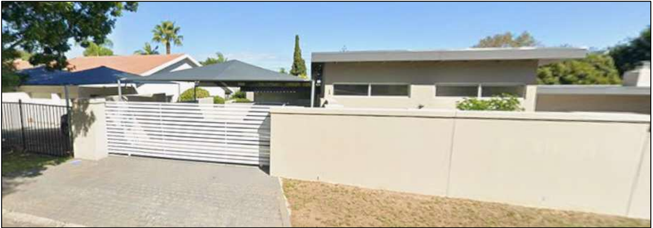
Figure 6: Similar situation with double shade port at no. 25 Tulbach road
