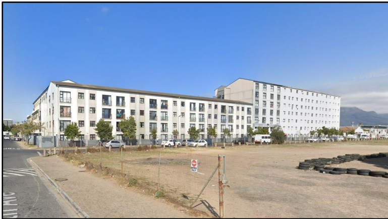
Figure 34 4 -7 storey apartments along Nyman Street
