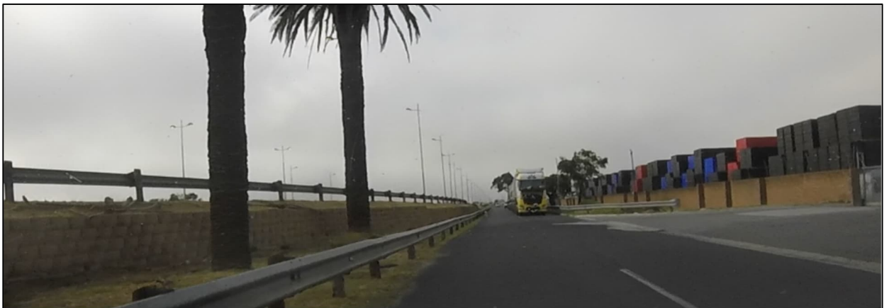
Figure A2: Heavy Vehicles obstruct Northbound Lane of Stranfontein Road (service road)
