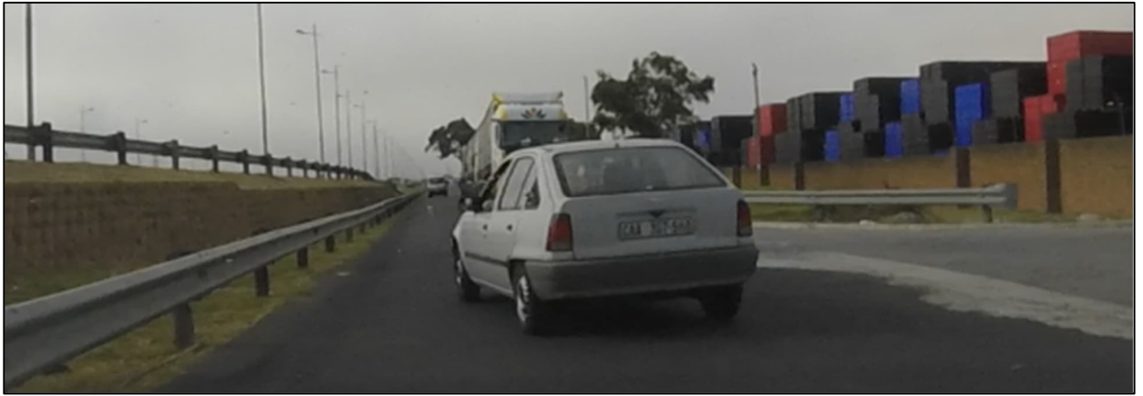
Figure A4: Northbound Traffic Travels in the Southbound Lane causing Conflict
