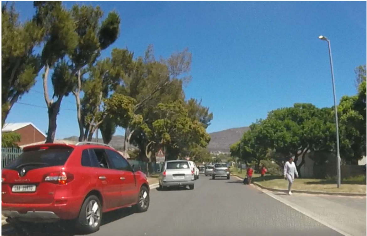
Figure A17: Raised Pedestrian Crossing in Corvette Avenue at Student Gate1 has no universal access or sidewalks.
