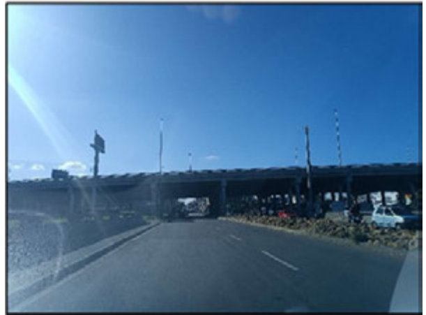
Figure 4. Intersection with M5 highway (captured 08/05/2024)
