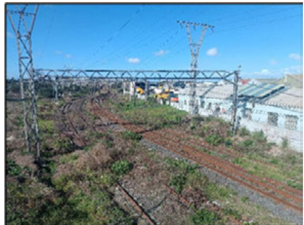
Figure 13. Central railway line (captured 08/05/2024)
